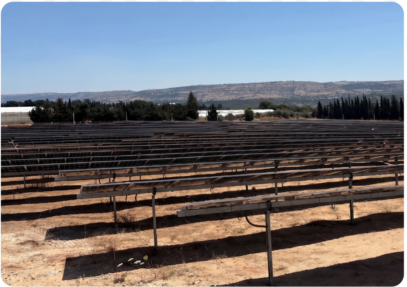
ILPAV SRL Plant
