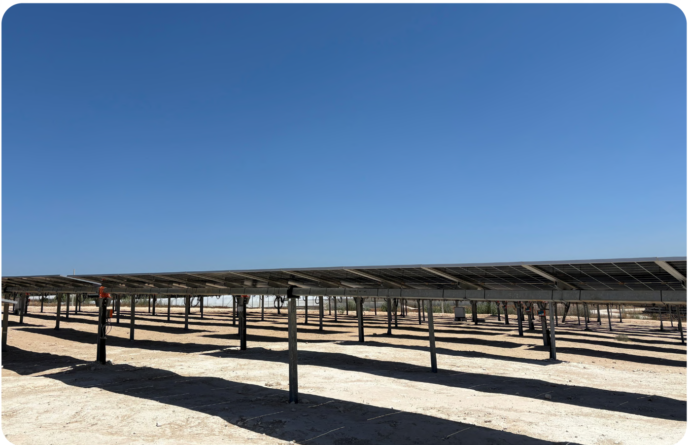
ILPAV SRL Plant
